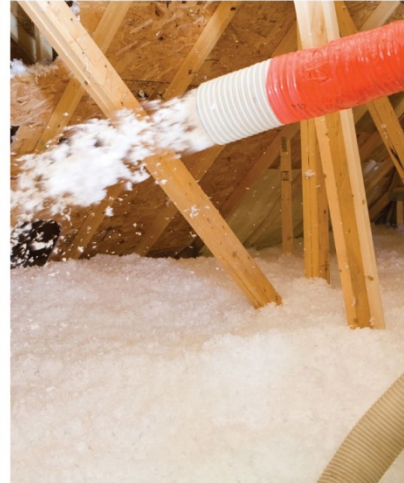
Attic insulation & air sealing
